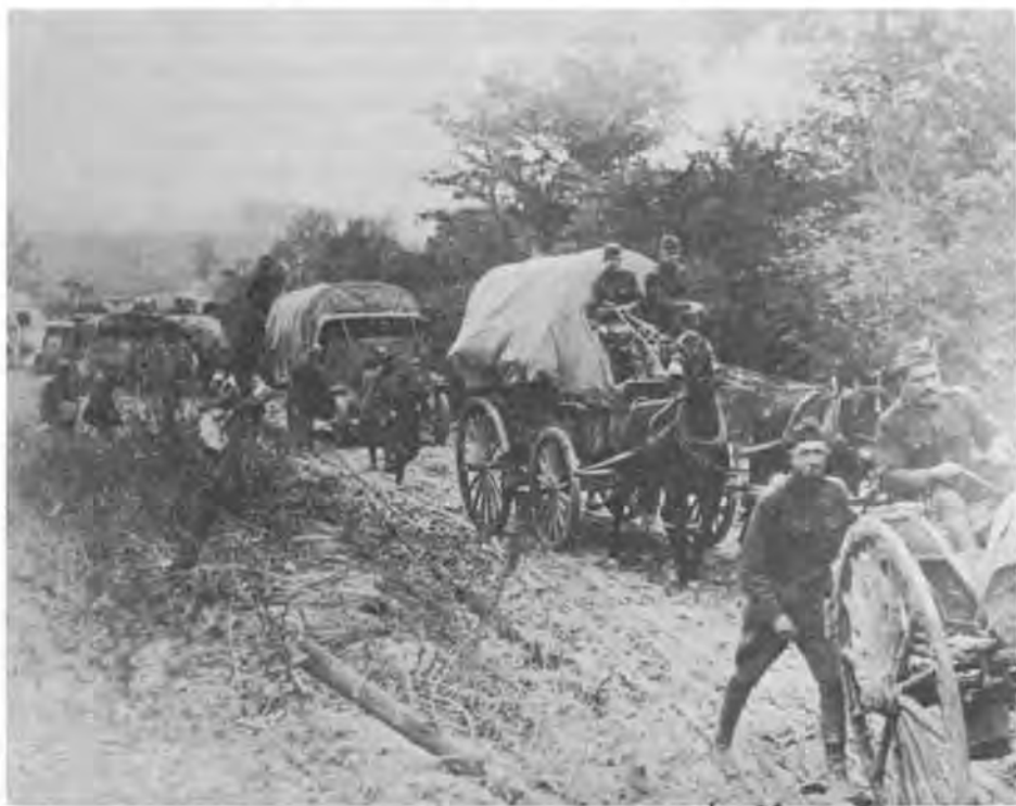
MOVING SUPPLIES TO THE FRONT, 1 OCTOBER 1918
