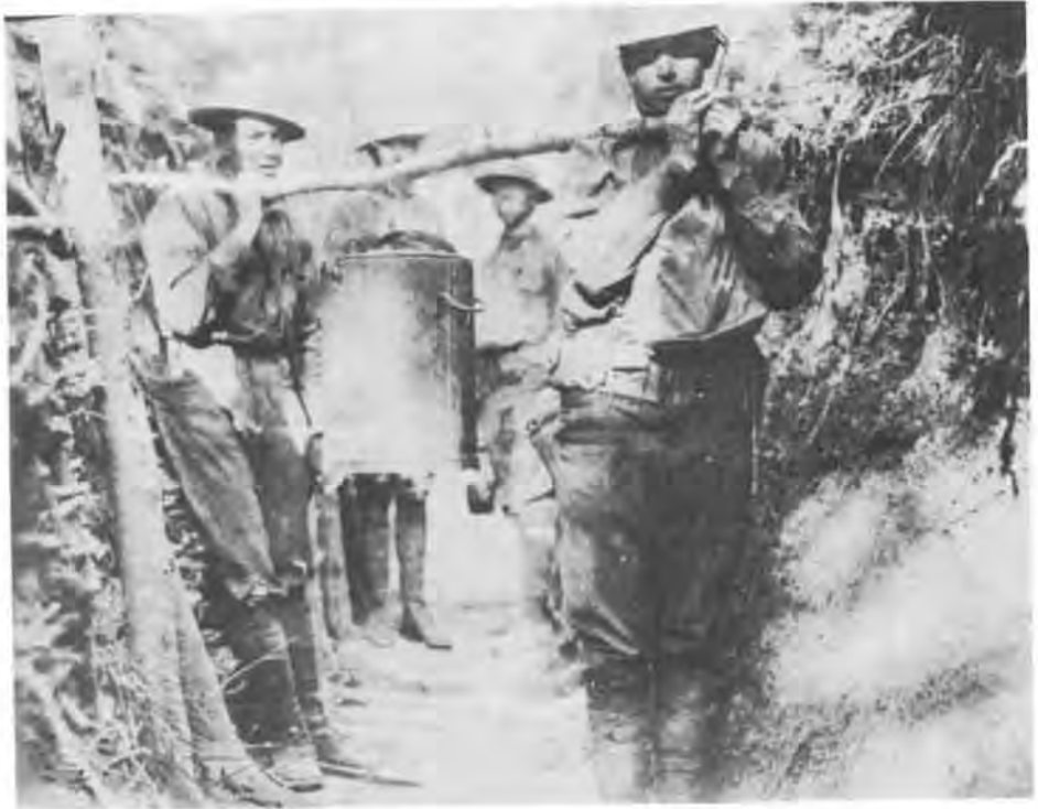
CARRYING FOOD TO MEN IN TRENCHES
